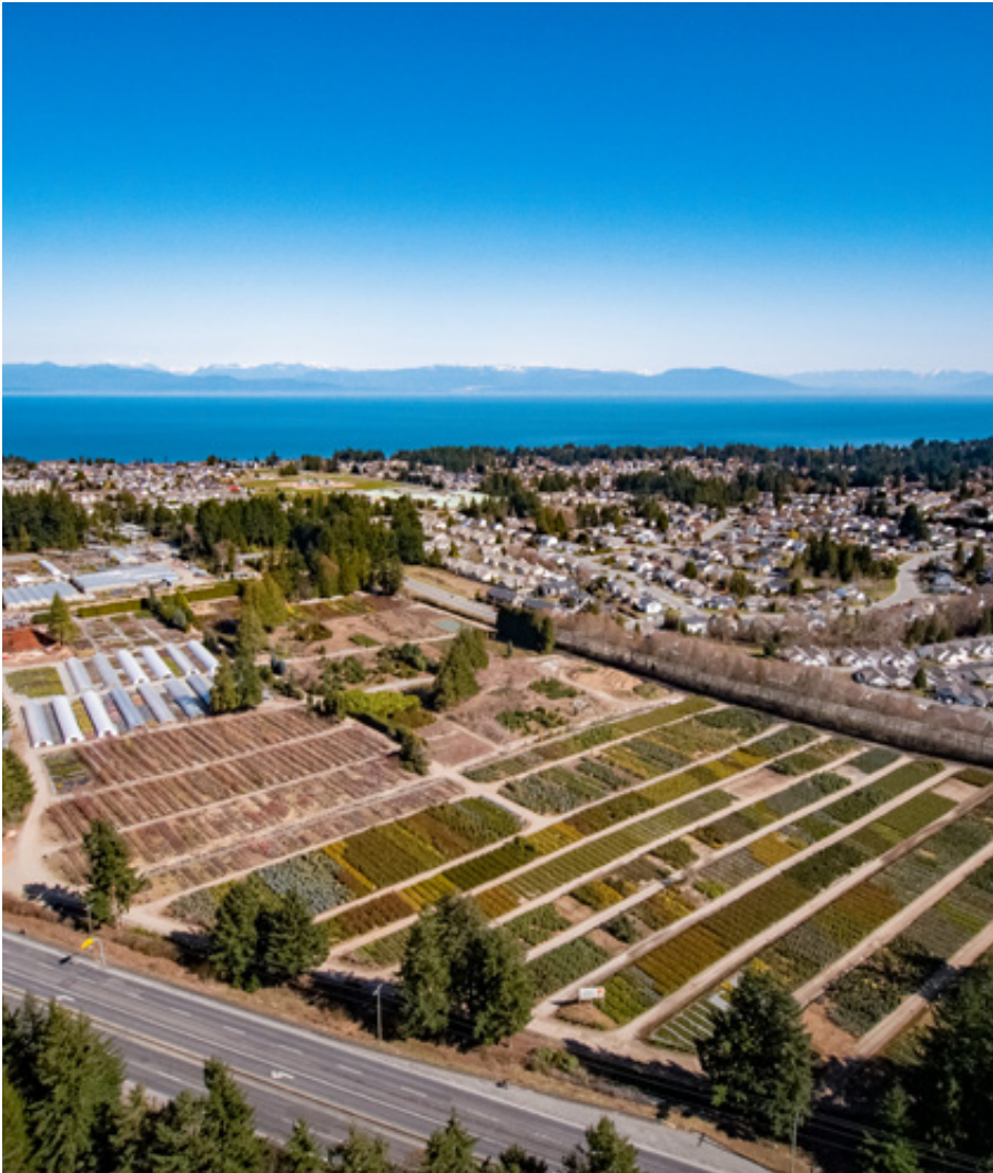
AERIAL VIEW OF SITE, LOOKING NORTHEAST
