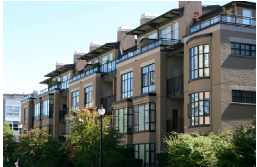
A building with a significant upper storey setback utilized as private balcony spaces
