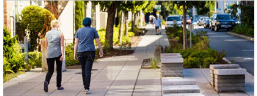
Sidewalk with integrated rain garden, street trees, and permeable paving
